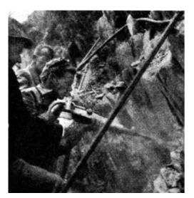
Figure 7: Swiss miner, 1930s, using a power drill.
